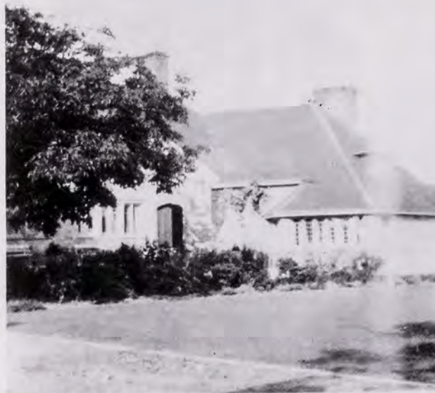
Fittleworth Mill: tennis court and house 1923.
