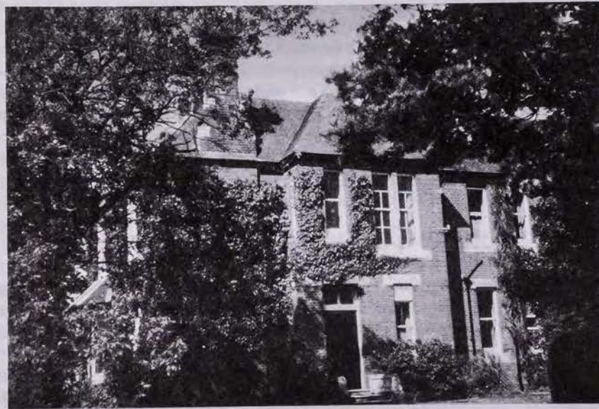
Red House in 1963. Courtesy of Mrs M. Manning.
