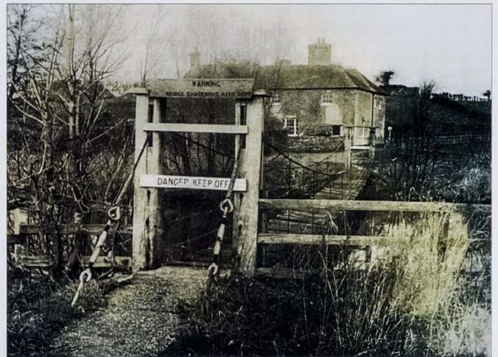
'Warning. Bridge dangerous. Keep off'. Rotherbridge, possibly in the early 1950s. Hungers Lane is just out of shot to the right. See 'Fatal Accident at Petworth' on page 47. Photographer unknown.
