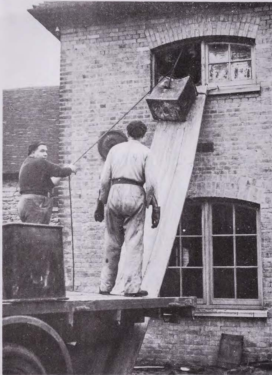
Dismantling the Battery House 1953. [Photograph by George Garland.]
