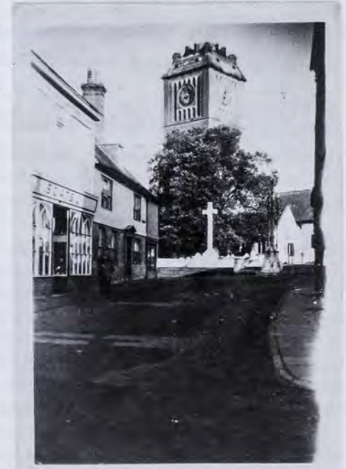
"The necessary work of demolition will be started any day now" said the Rector. By the time this snapshot was taken in October 1948 the steeple was already only a memory.
