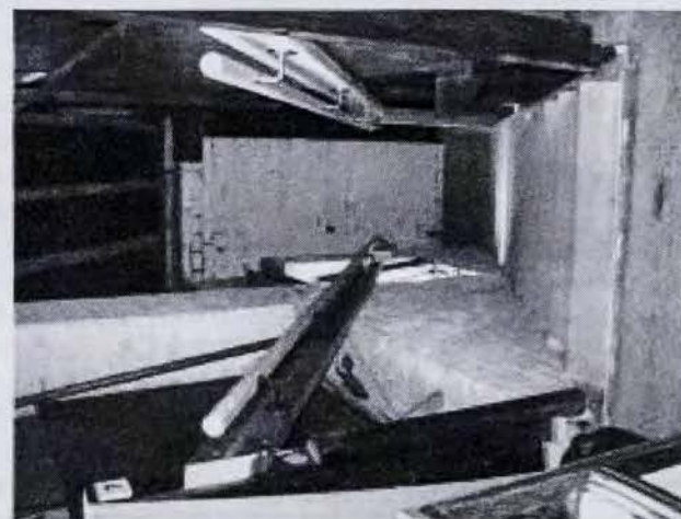
New Stair case in Pump House
