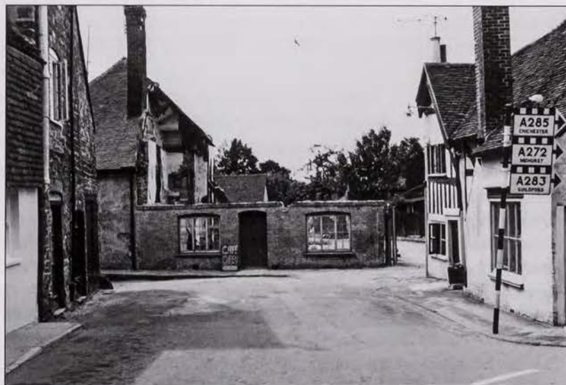
Damer's Bridge 1960, preparing the entrance to the new Car Park.
