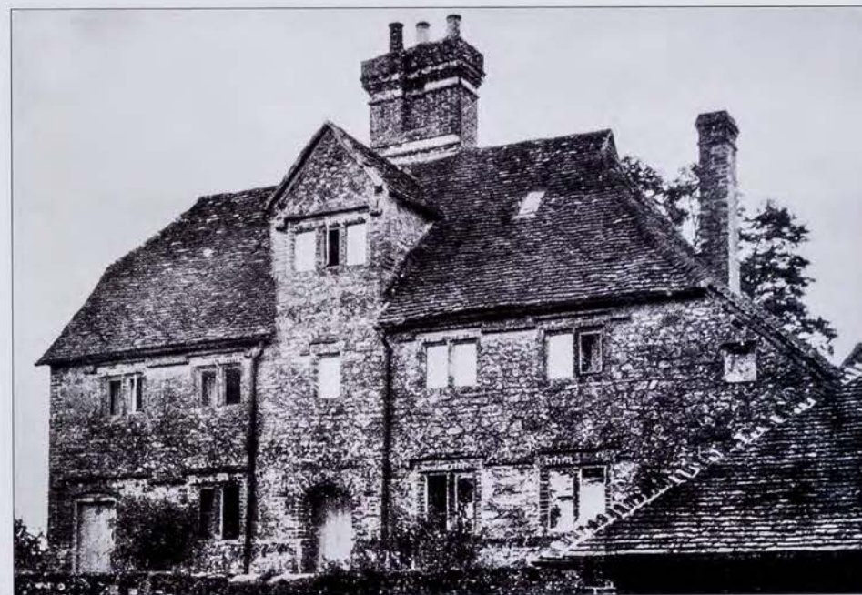
ABOVE Coxland in the early 1930s. At this time, towards the end of its life, the 'grand old house' had been divided into two, or possibly more, 'cottages'. This is suggested by the door on the extreme left with its tell-tale estate number and which is clearly an insertion replacing an earlier window. The house was stylistically very similar to Coates Manor a few miles away which dates from the early seventeenth century and which was once known as No. 24 Leconfield Estate.
