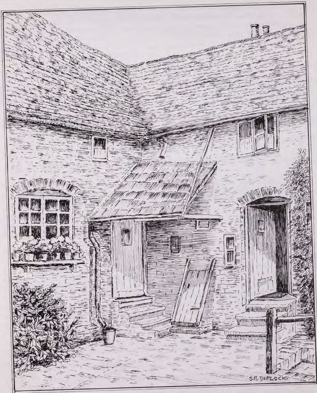
A rear view of cottages in North Street. This illustration has been redrawn by Rendle Diplock after an original water-colour owned by Peter Wakeford and dated 1918.
