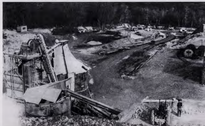
A Garland photograph of Duncton quarry c.1951. The primary crusher is in the foreground while the kiln loading area can be seen in the centre.
