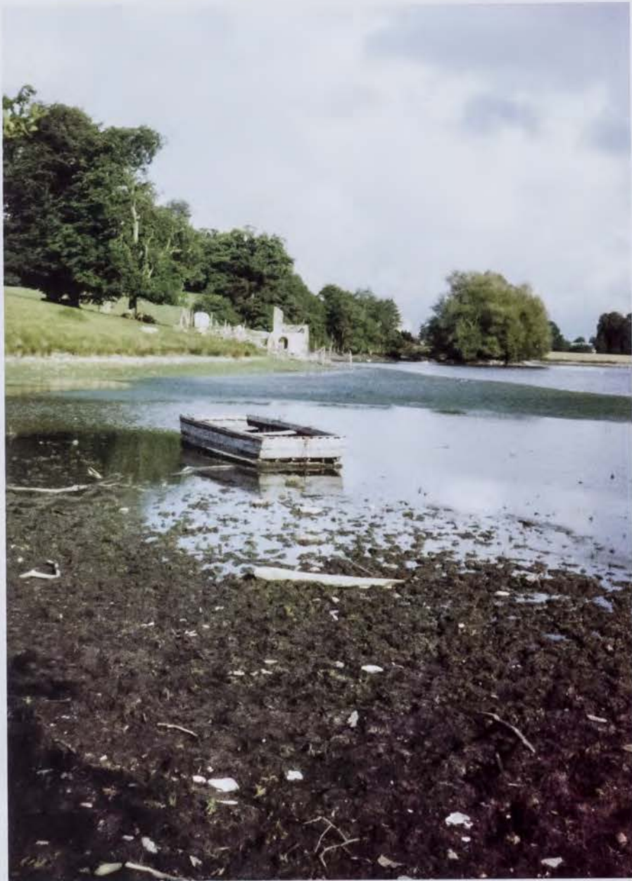
Draining and restoration of the Upper Lake, Petworth Park 1983. Lord Leconfield's punt has surfaced; it was used for shooting parties on the river. Note repairs to the boat house. See "Delicate balances."
