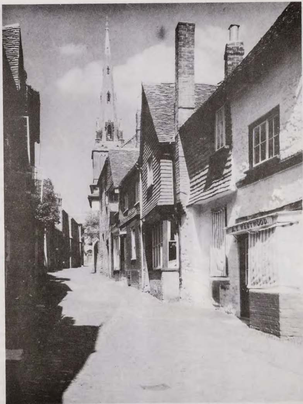
"I can never come up Station Road, ..... without thinking what a great loss the steeple was to Petworth." This photograph was taken an hour before demolition work began in 1947.
