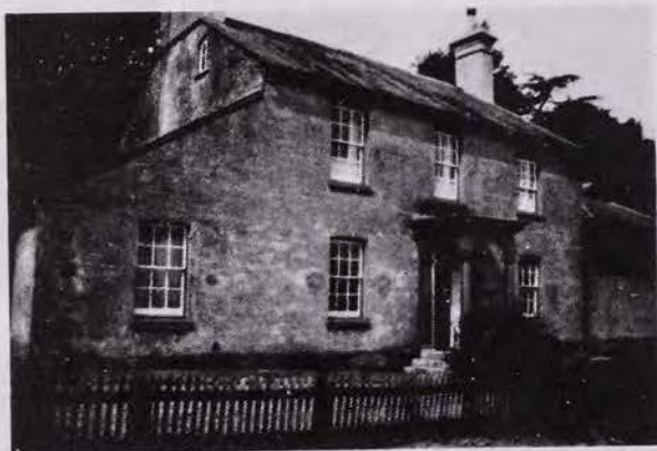
The Butler's Cottage, North Street. 1931.
