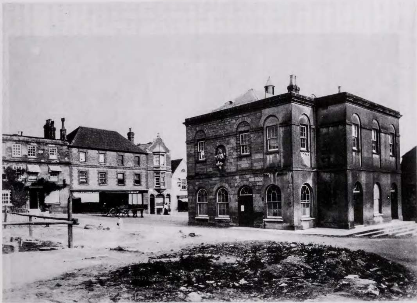
Petworth Town Hall - North and West elevations 1900. Photograph by Walter Kevis.
