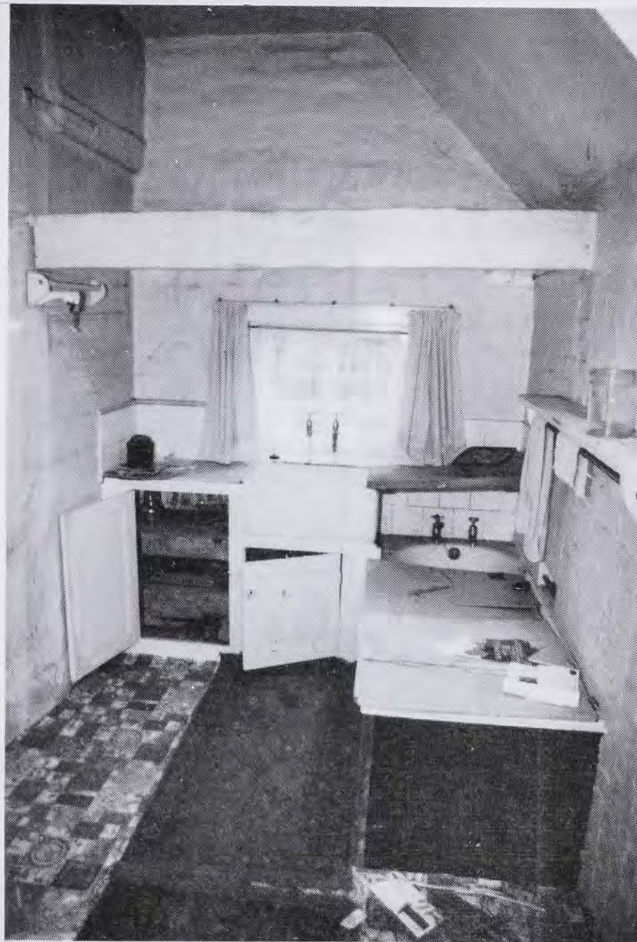
The scullery at 346 High Street. Photograph by Barry Norman.
