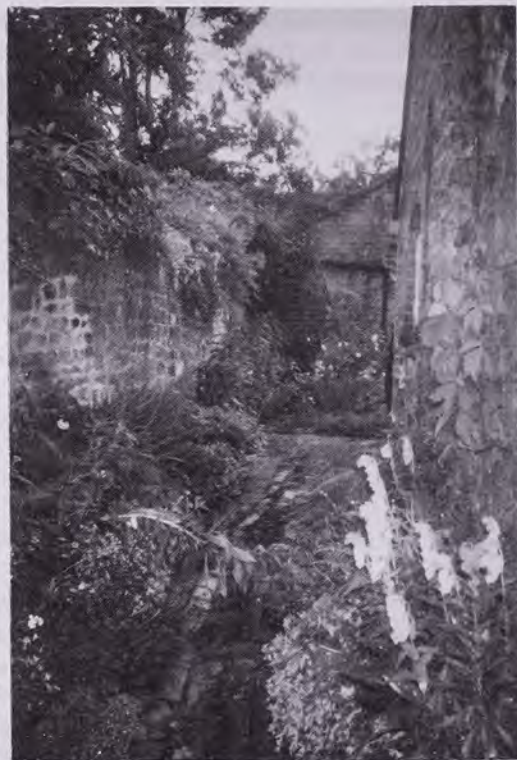
Entrance to 346 High Street after heavy rain. 1999.
